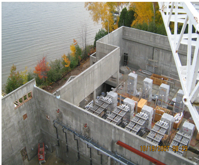
Installation of Pall Membrane Racks October 2007
