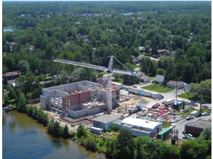
Water Treatment Plant Construction Site July 2007
