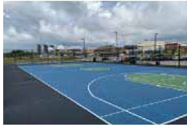
Outdoor Multi-Use Recreation Courts (2021)
